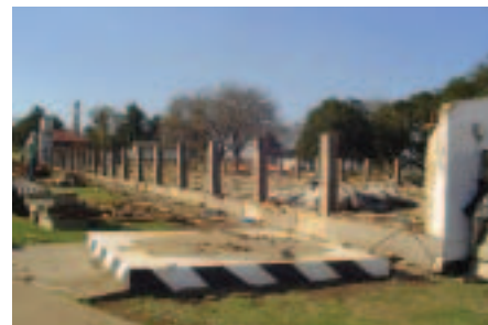
Demolition of old broiler houses
